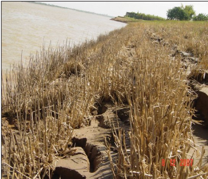
Photo 20: Upper and lower: alluvial silt deposit between vetiver rows on lower part of the slope.
