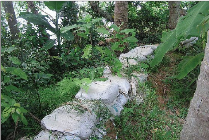
Photo 12: Upper: severely eroded bank of the Tra Khuc River, at Binh Thoi Commune; lower: primitive sand bag protection.
