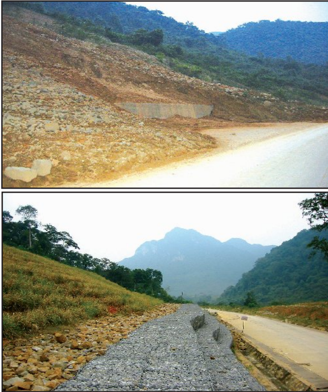
Photo 27: Da Deo Pass, Quang Binh: Upper: Vegetation cover is destroyed, revealing ugly and continuous failures of cut slopes; lower: Vetiver rows on top of the slope very slowly squeeze down, considerably reducing the failed mass.
