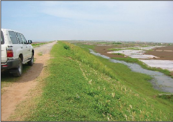
Photo 24: In North Vietnam; Upper: Vetiver planted on outer side of a newly built sea dike in Nam Dinh province; lower: on the inner side of the dike, planted by the local Dike Department.
