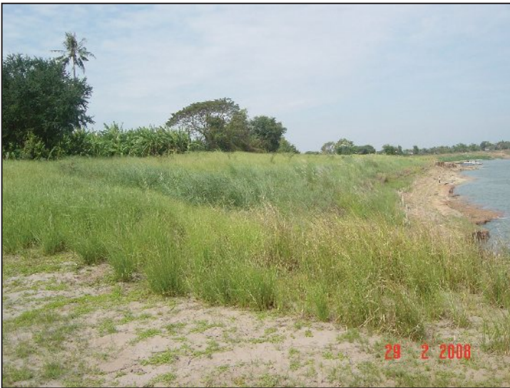
Photo 21: Fully recovered after the flood (upper) and new planting on the bare lower section of slope (lower).
