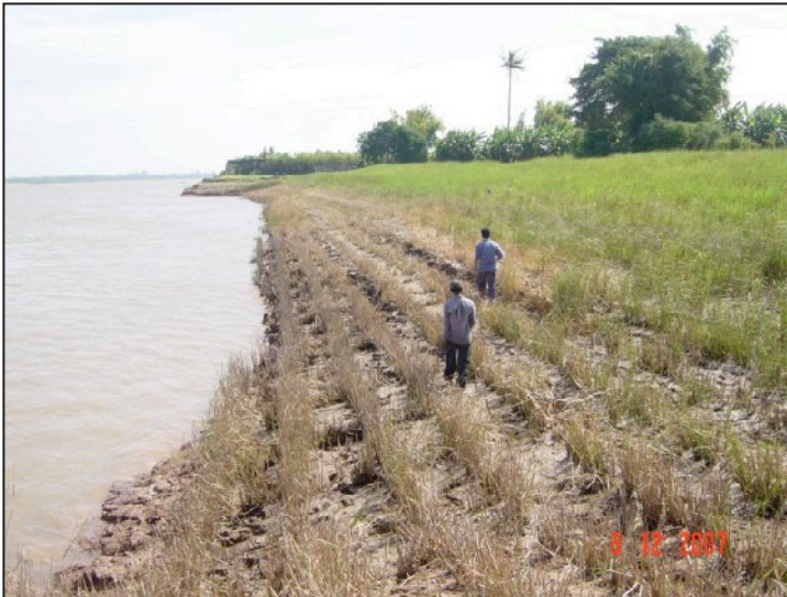
Photo 18: Flood water started coming up (upper); and dead looking vetiver on lower slope after water retreats (lower).
