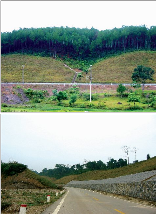
Photo 25: Upper: Vetiver stabilizes cut slopes along the Ho Chi Minh Highway; lower: both alone and in combination with traditional measures.
