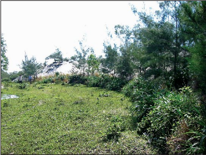
Photo 6: Upper: Vetiver protects bridge abutment along National Highway nr.1; lower: December 2004, local species have replaced vetiver.
